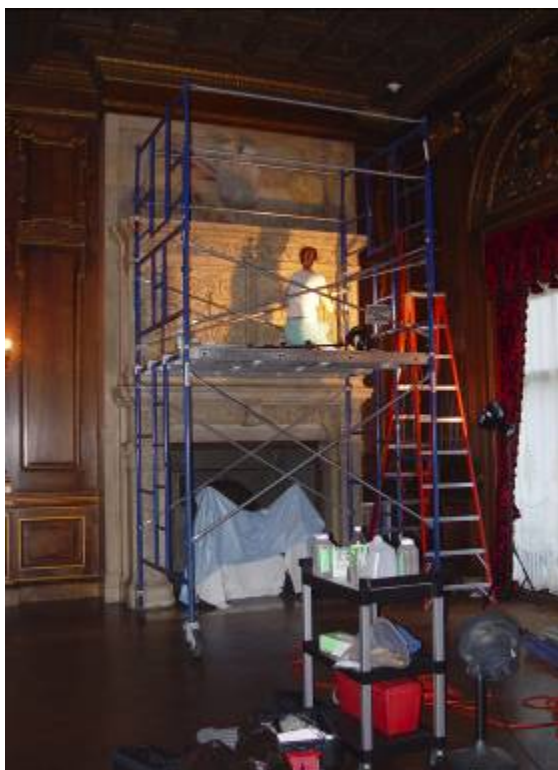
20. Conservator Cleaning Stone Overmantel, Vanderbilt Mansion, Hyde Park, NY.
