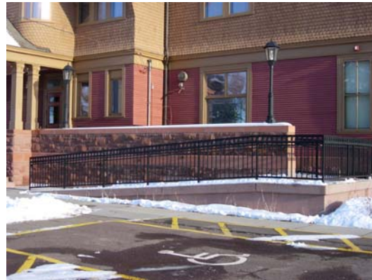
44. Fairlawn Mansion, Superior, WI. Left to Right: Retractable Sprinkler Head in Ceiling, Wheelchair Ramp. The staff at Fairlawn Mansion achieved resource protection and visitor access goals through good planning and design. Retractable sprinkler heads are virtually unnoticeable to the visitor. The scale, materials, and design of the exterior wheelchair ramp provide access without detracting from the house's guest entrance.
