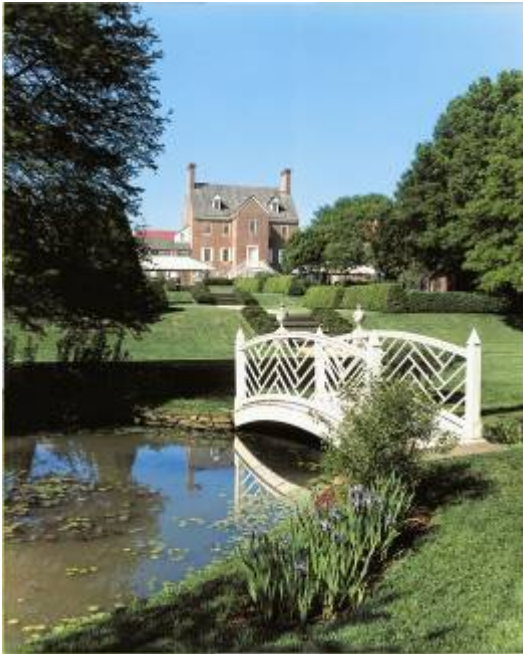
2. William Paca House and Garden, Annapolis, MD. According to the Secretary's Standards , William Paca House and Garden's landscape, structure, and historic furnished interior are all considered restoration projects. While applying the same treatment to all resources at one property is the ideal, it is the exception rather than the rule because different resources survive into the present with different degrees of integrity.
