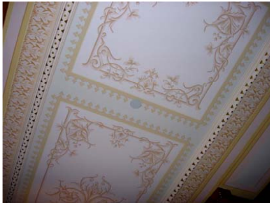
44. Fairlawn Mansion, Superior, WI. Left to Right: Retractable Sprinkler Head in Ceiling, Wheelchair Ramp. The staff at Fairlawn Mansion achieved resource protection and visitor access goals through good planning and design. Retractable sprinkler heads are virtually unnoticeable to the visitor. The scale, materials, and design of the exterior wheelchair ramp provide access without detracting from the house's guest entrance.
