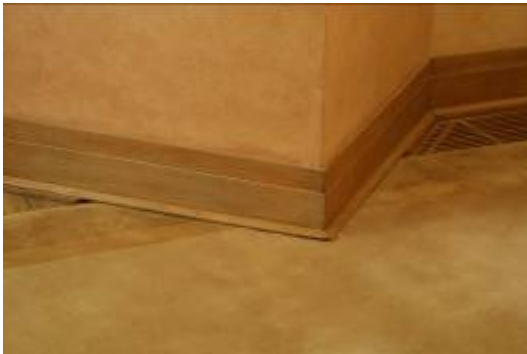
7. Living Room and Living Room Detail, Purcell-Cutts House, Minneapolis, MN. At times a building can dictate where furnishings are located such as the placement of a watchmaker's workbench near a window (not shown). Rarer is a furnishing affecting a building's construction. Here a space under a corner accommodates a large area rug.
