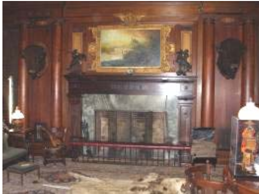
10. North Room, Sagamore Hill, Oyster Bay, NY. The mounted buffalo heads flanking the fireplace are character-defining features. Their removal would greatly diminish the room's historic character.
